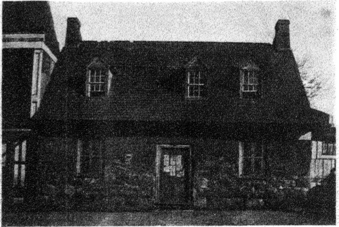
OLD STONE HOUSE, BUILT IN 1737.
