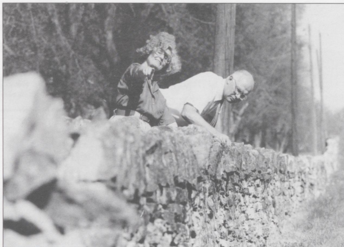
Carolyn Murray-Wooley and Karl Raitz examine a level coursed dry-laid rock fence near the Kentucky Horse Center off Paris Pike.
