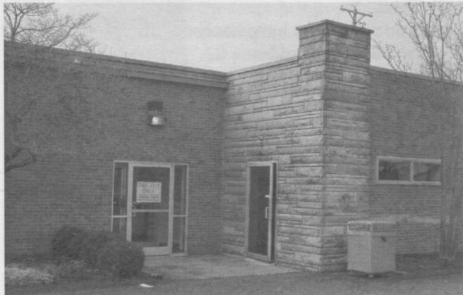
This building at 913 Georgetown Road was built in the early 1960s to be Holiday Lanes, the first integrated bowling alley in Lexington. It has been owned by the city since 1980 and now used by the Community Action Council. Tom Eblen teblen@herald-leader.com
