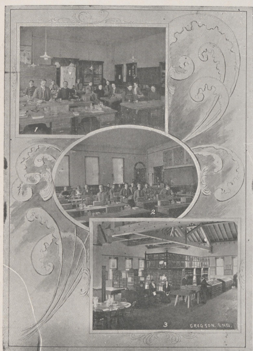
Interior Views, Natural Science Building.
