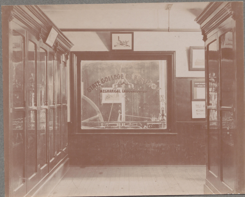
MECHANICAL HALL ENTRANCE TO MECHANICAL LABORATORIES
