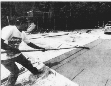
SMOOTH WALKING Fred White works on a sidewalk at the foot of the Finkbeiner Building, one of several UK renovation projects.
