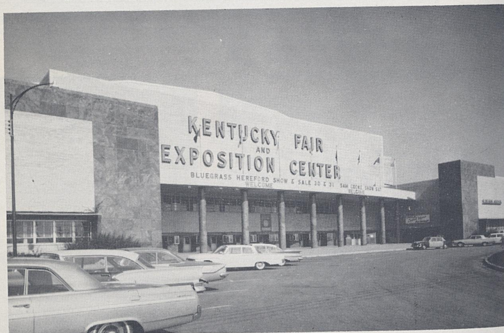
The Kentucky Fair and Exposition Center, Louisville, is site of Kentucky State Fair, numerous national conventions, athletic events, and entertainers. The grounds also include a football stadium, two-high exhibition wings, meeting rooms, dining room, golf course, and an auto race track.
