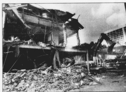
The old civil engineering building, located on the south side of the Engineering Quadrangle, will be replaced within two years by an $11.6 million facility.
