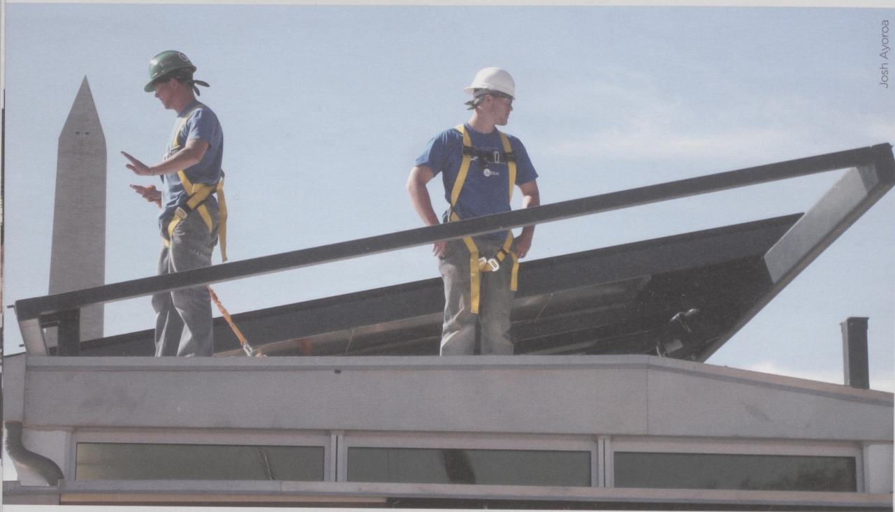
Ross Graham (left) and Chad Gallas await the placement of the last PV panel. The rooftop array not only generates power, but also shades and cools the roof.
