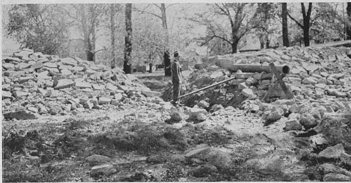
Both these dams failed because of faulty construction. That at the left settled too much at one point and then washed out; that at the right was destroyed by overflow when the spillway, built too small, failed to carry off the surplus water.
