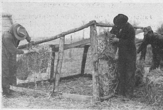
Constructing walls of straw
