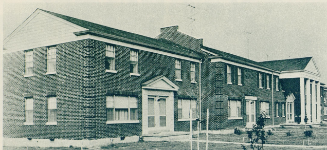
This is one of the new Wherry housing units at Fort Campbell. These apartments will house military personnel.
