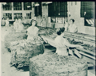
Workers at left remove the tobacco from the hogsheads after it has been taken from the vacuum units. Above, women workers are shown blending various grades of tobacco. The blended tobacco is carried to the next process on a conveyor belt.
