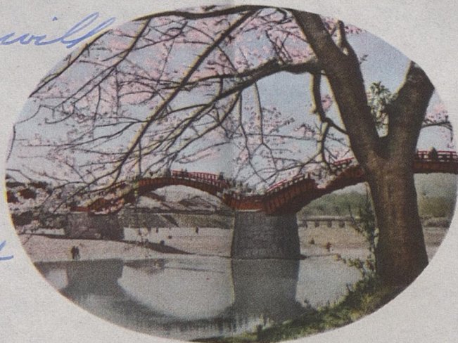
Kintai-Bridge at Iwakuni
