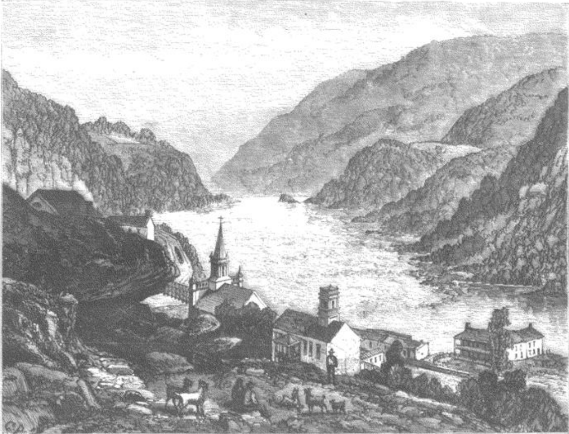
View from Jefferson Rock.
