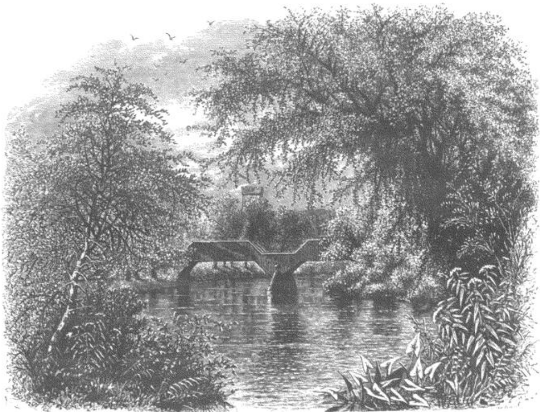
Whipple's Bridge on Blackstone River.
