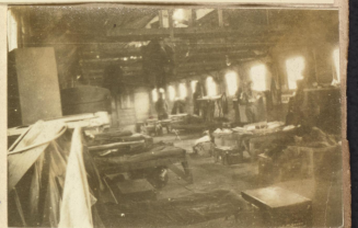
Gas House inside
