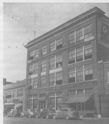
The four-story building on the right is 249-255 East Main Street (Lexington), now occupied by Portofino Restaurant on a portion of the ground floor and by Thomas and King offices in the remainder of the building. The two-story building on the left is 243-247 East Main Street, which was later demolished and is now the location of a surface parking lot. Judging from the appearance of the cars on the street, the photo was taken between 1928 and 1945. (Thanks to Hanna Smith, Bruce Naude, Mike Ades, and Jason Flahardy for providing this information.)
