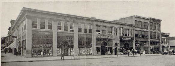
THE HOME OF THE COMMERCIAL CLUB OF ASHLAND
