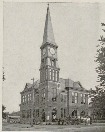
FIRE DEPARTMENT NO. 1
