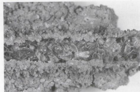
Dead termites packed inside a foraging tunnel in a crawl space under a house following an exterior termite treatment
