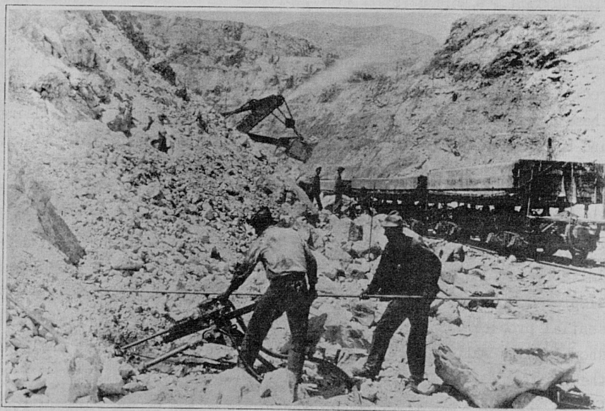
FIGURE 23.— TOE-HOLE DRILLING AT AN OPEN-CUT COPPER MINE
