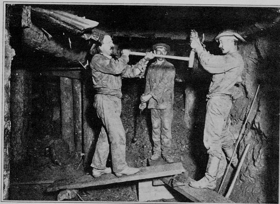
FIGURE 3.— DOUBLE-JACKING UNDERGROUND
