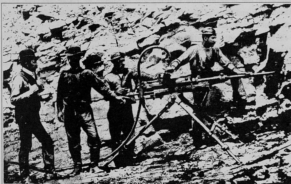
FIGURE 17.— EARLY PISTON DRILL IN A QUARRY
