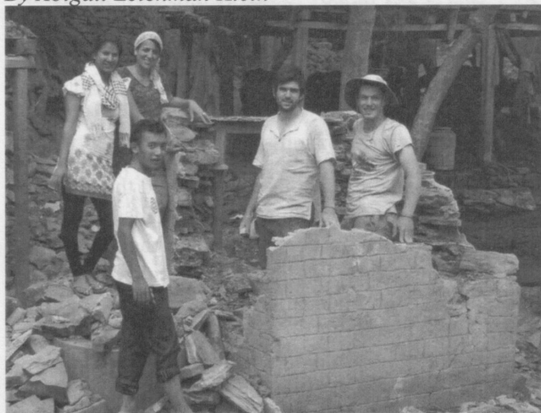
How several Israeli professionals are giving Nepal villagers tools to rebuild their houses and their lives after the earthquakes.
